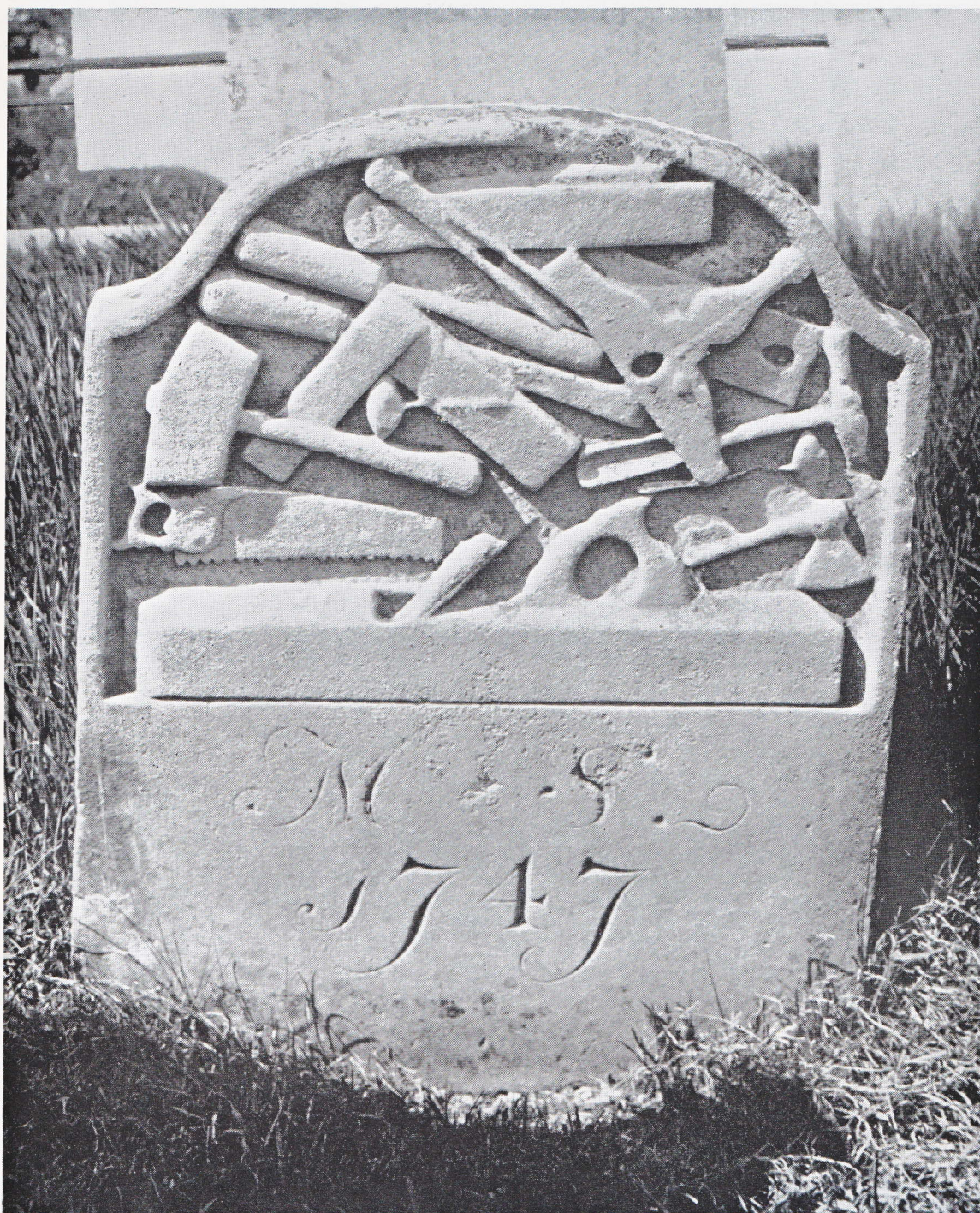
35. The earliest dated evidence of a closed handsaw handle. A carpenter's gravestone in the churchyard of St John-sub-Castro, Lewes, Sussex, 1747
