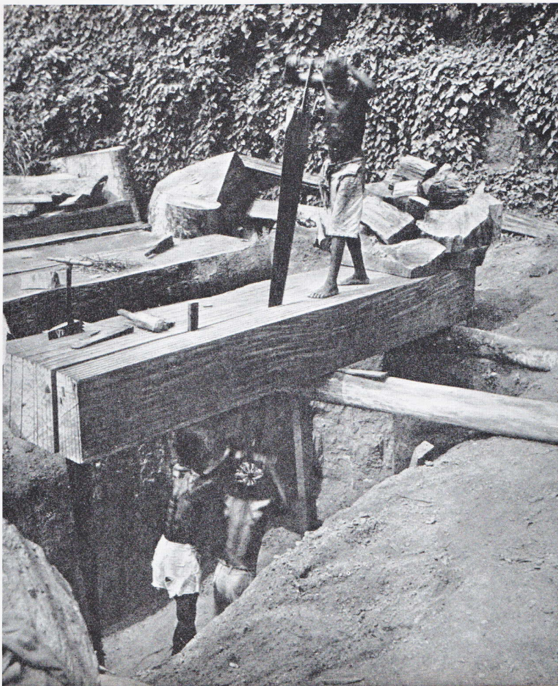
66. Pit-sawing in Ghana. Saws up to ten feet long are used frequently
