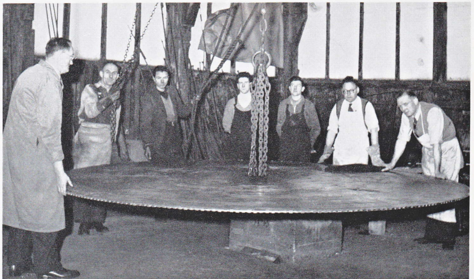
87. A Spear and Jackson team of three smithers prepares to tension the largest saw ever made
